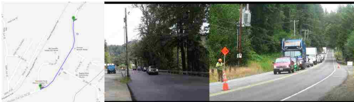
FIGURE A-5 Location and site photos for work zone #5
