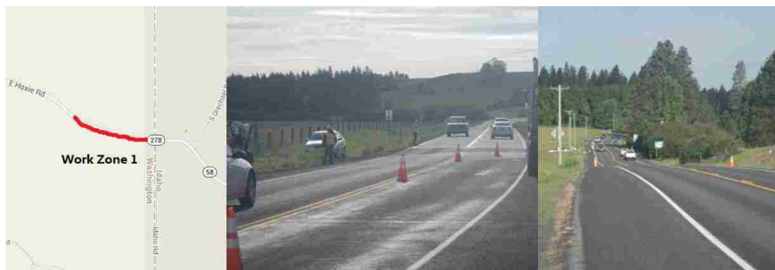
FIGURE A-1 Location and site photos for work zone #1
